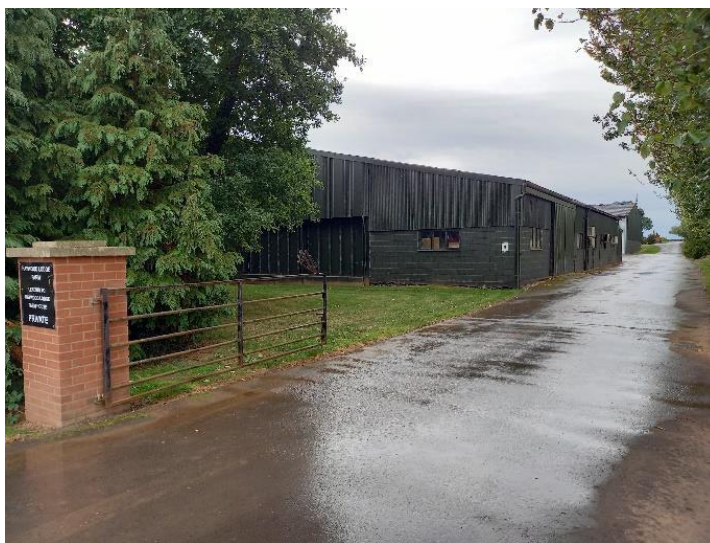
Vast road side frontage, access and driveway to the new Haywood Lodge Farm House and commercial buildings set in 'the group' separating The Granary from the Cottages and recalibrating the reading of the farmstead.
